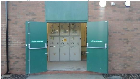
Figure 4 View of Three Panel 33kV Switchgear
