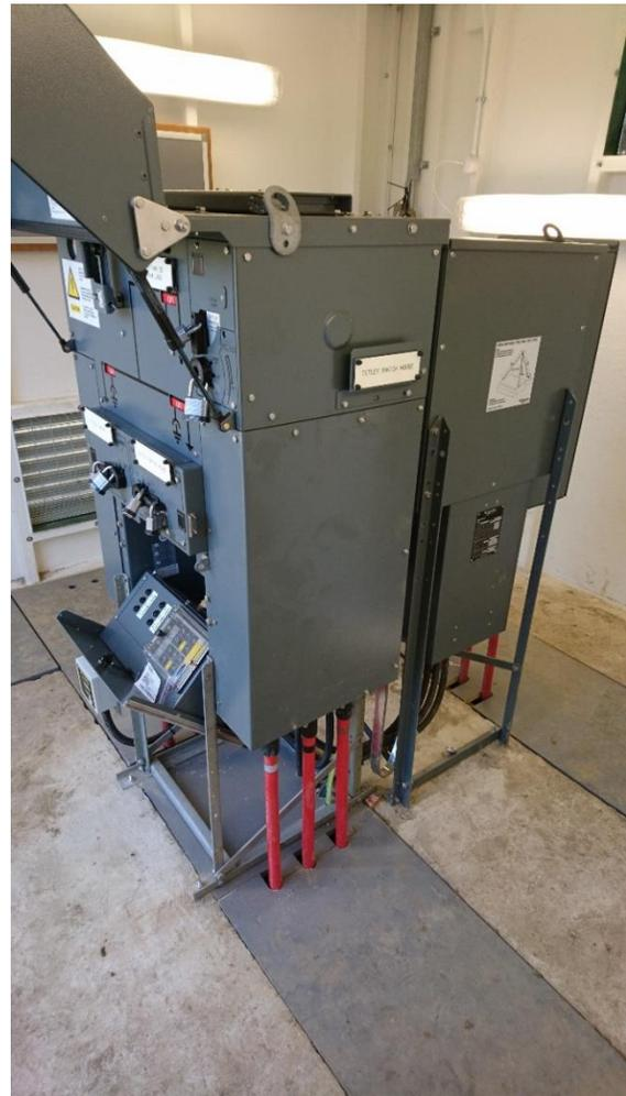
Figure 8 Metering RMU at Eaglescliffe
