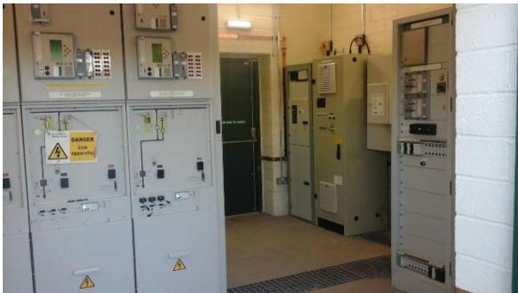
Figure 5 Interior of 33kV Substation Showing Various Apparatus
